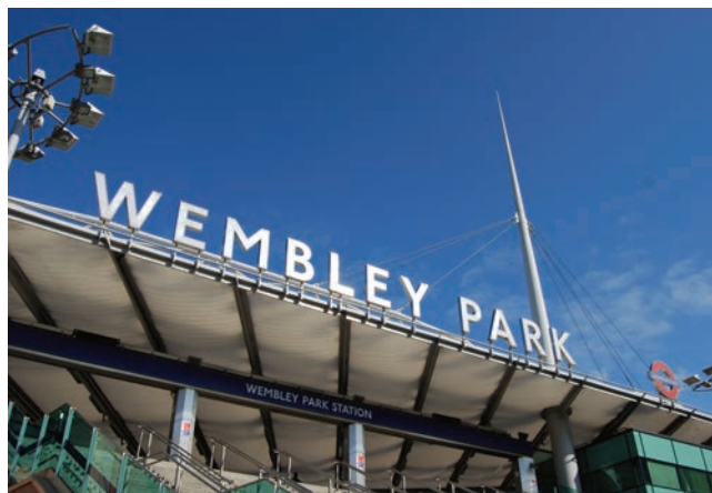
Picture 4.29 Wembley Park Station
