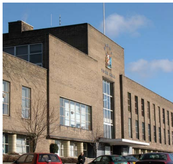
Picture 4.6 Brent Town Hall (Grade II)
