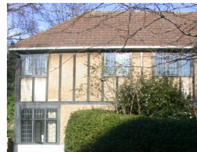
Simple half timbering to the first floor
