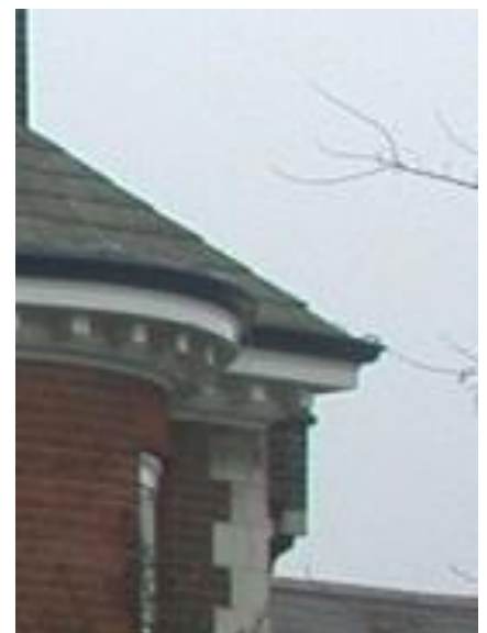
Dentiled Eaves at 810 Harrow Road
