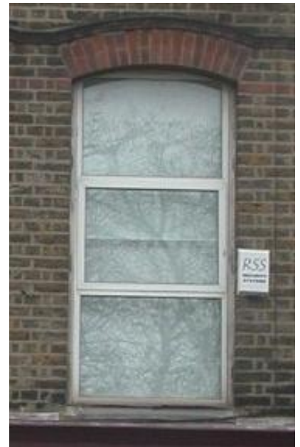
Inappropriate Window Replacement 792 Harrow Road
