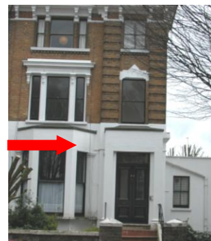
Cornice and capital details to the windows removed
