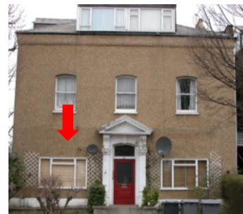
Original windows removed, original brickwork rendered over and dormers added
