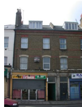
Neasden Lane North
