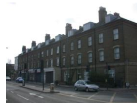
Neasden Lane North
