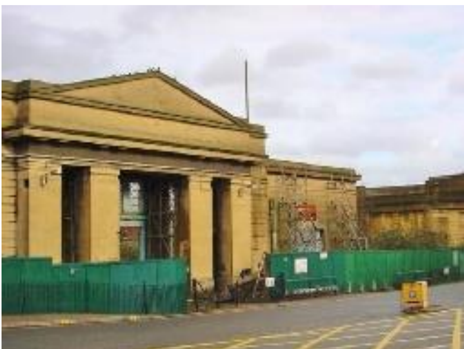
The Palace of Arts building awaiting demolition, November 2002.
