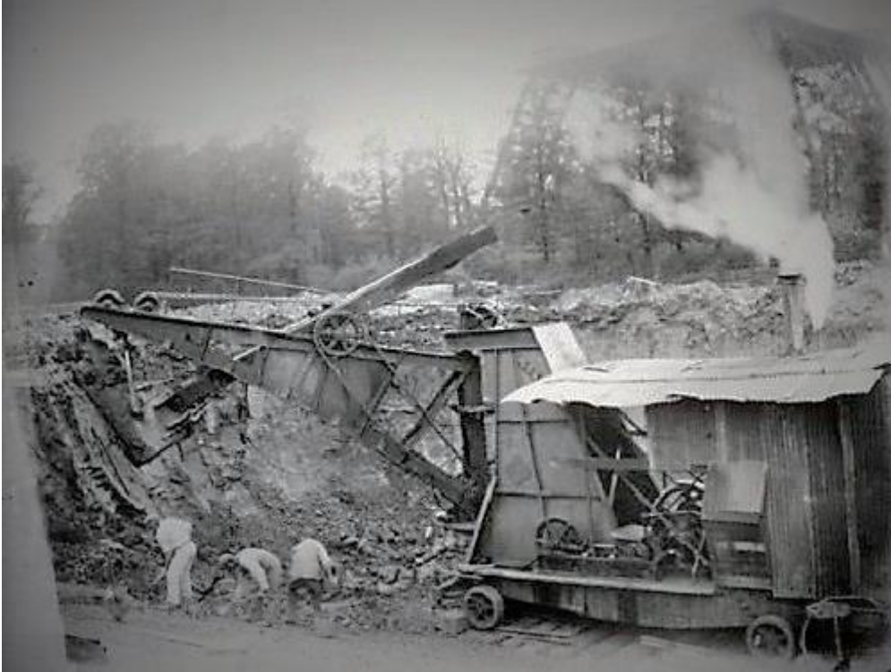
11. The Great Central Railway branch line under construction, c.1903. (Brent Archives online image 9253)
