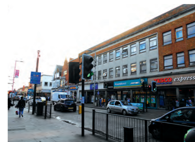
Site of Mark's and Spencer's 2019
