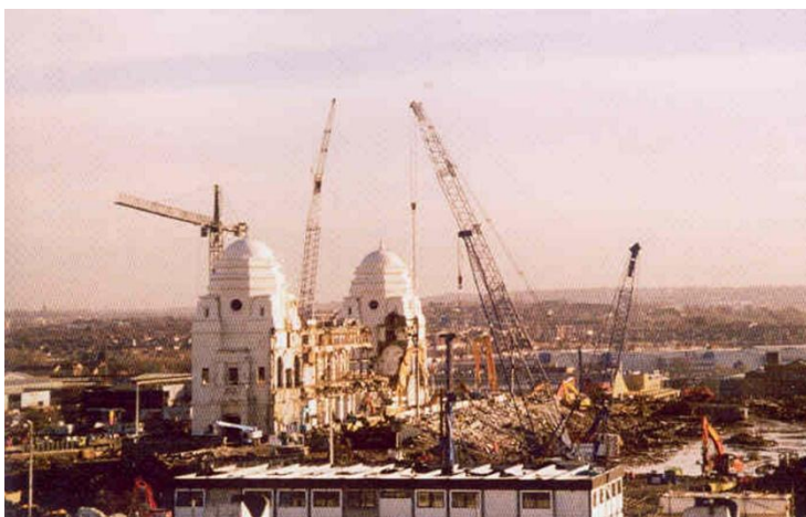
Demolishing the old Stadium, January 2003.
